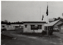
The headquarters building at Butterworth
